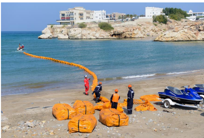
Figure 1. Deployment of booms around oil spills in Oman (source: Oman's Environment Authority).
